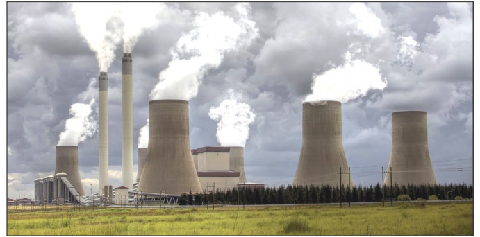
Coal Fired Power Station, South Africa
